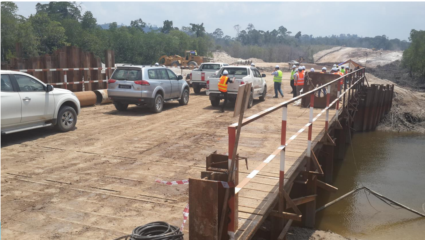
Temporary bridge at Sg. Belinsah built to transport materials across
