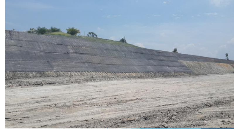
Slope protection by covered hydroseeding
