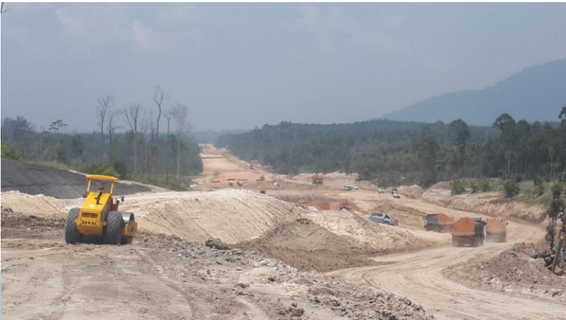
Panoramic view of Telok Melano-Sematan Roadworks in progress
