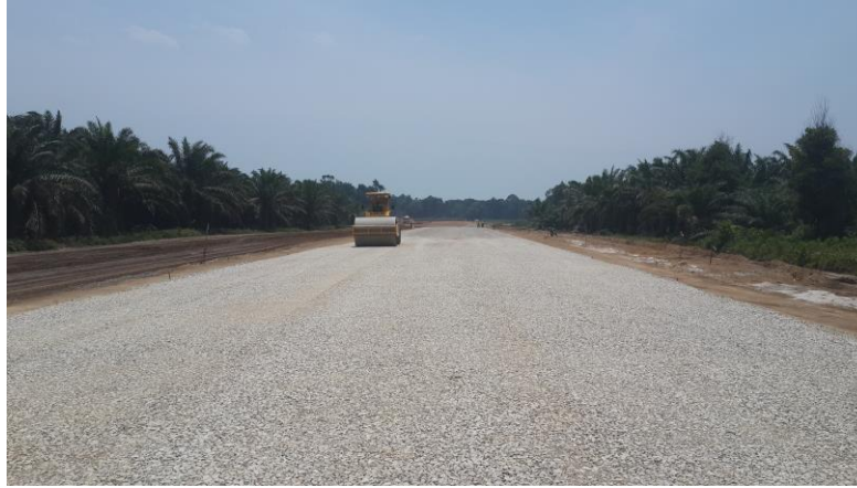
Laying of Sub-Base in progress
