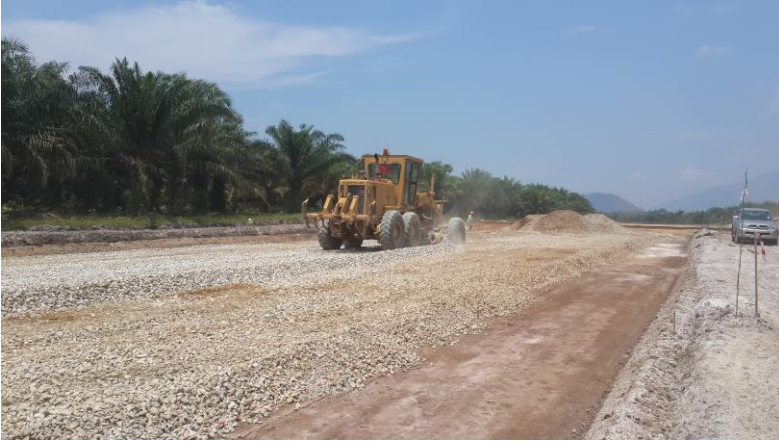
Laying of Sub-Base in progress
